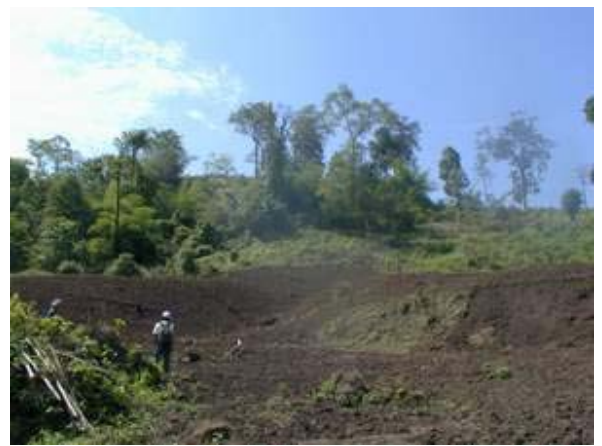
4. Penstock Slope from P/H
