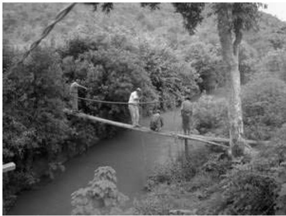
1. Discharge Measurement at the Intake Site
