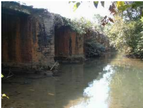
1. Existing Bridge near Intake Site
