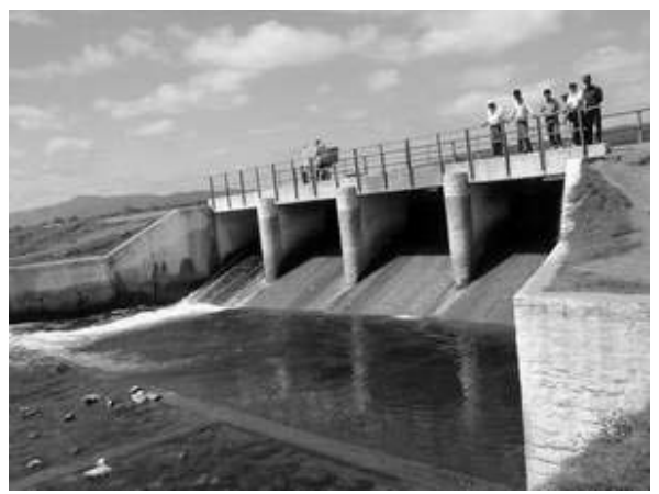
2. Outflow from Heho Dam
