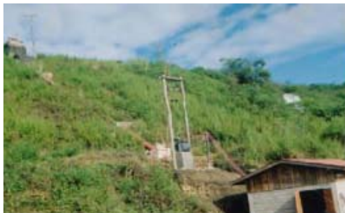
Penstock and Distribution Line
