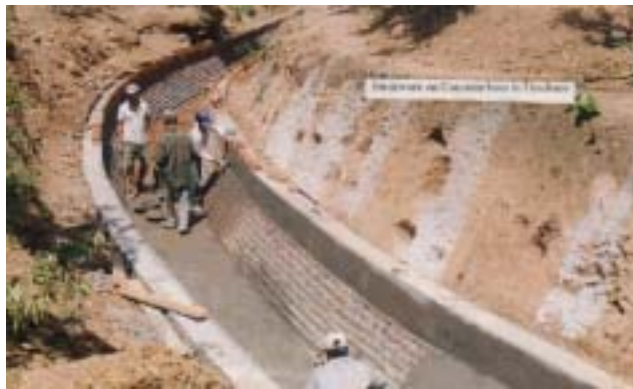
Stone Masonry Canal, Sempai
