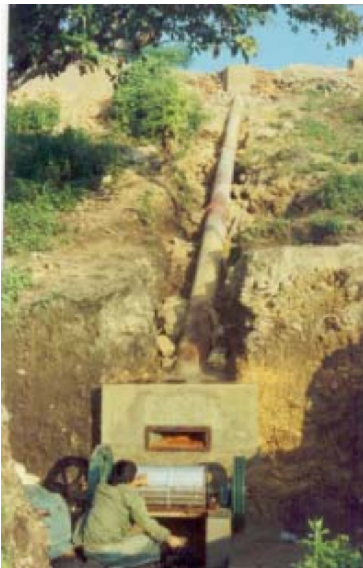
Construction on Self-Help: Waterways - Penstock (Pressure Pipe)
