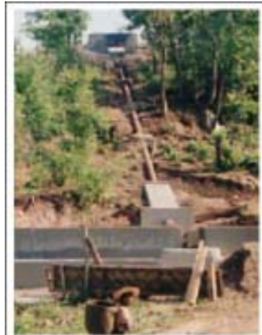
Anchor Block of Penstock
