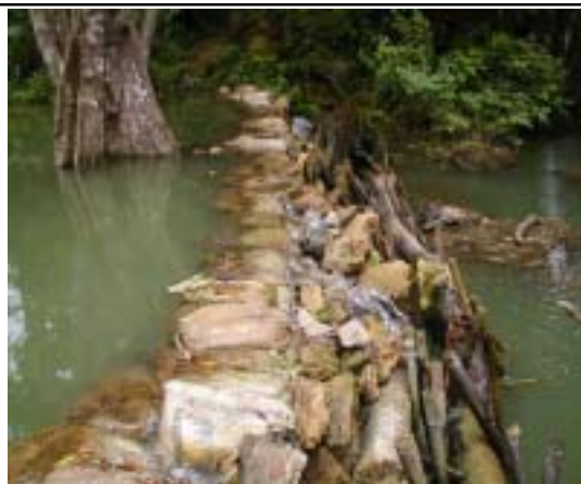
Sample of weir by sandbags
