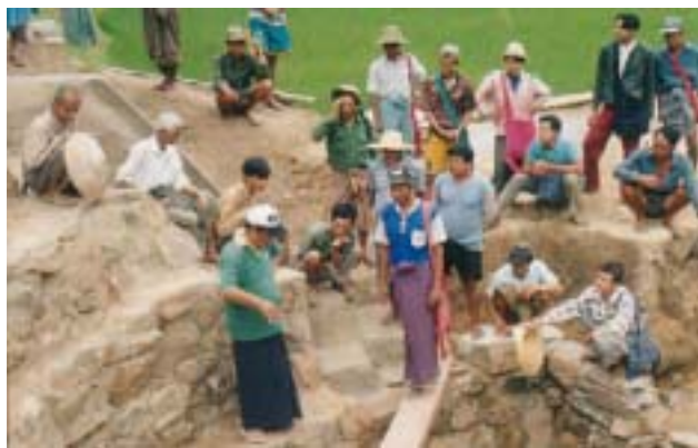
Construction on Self-Help: Waterways - Power Canal
