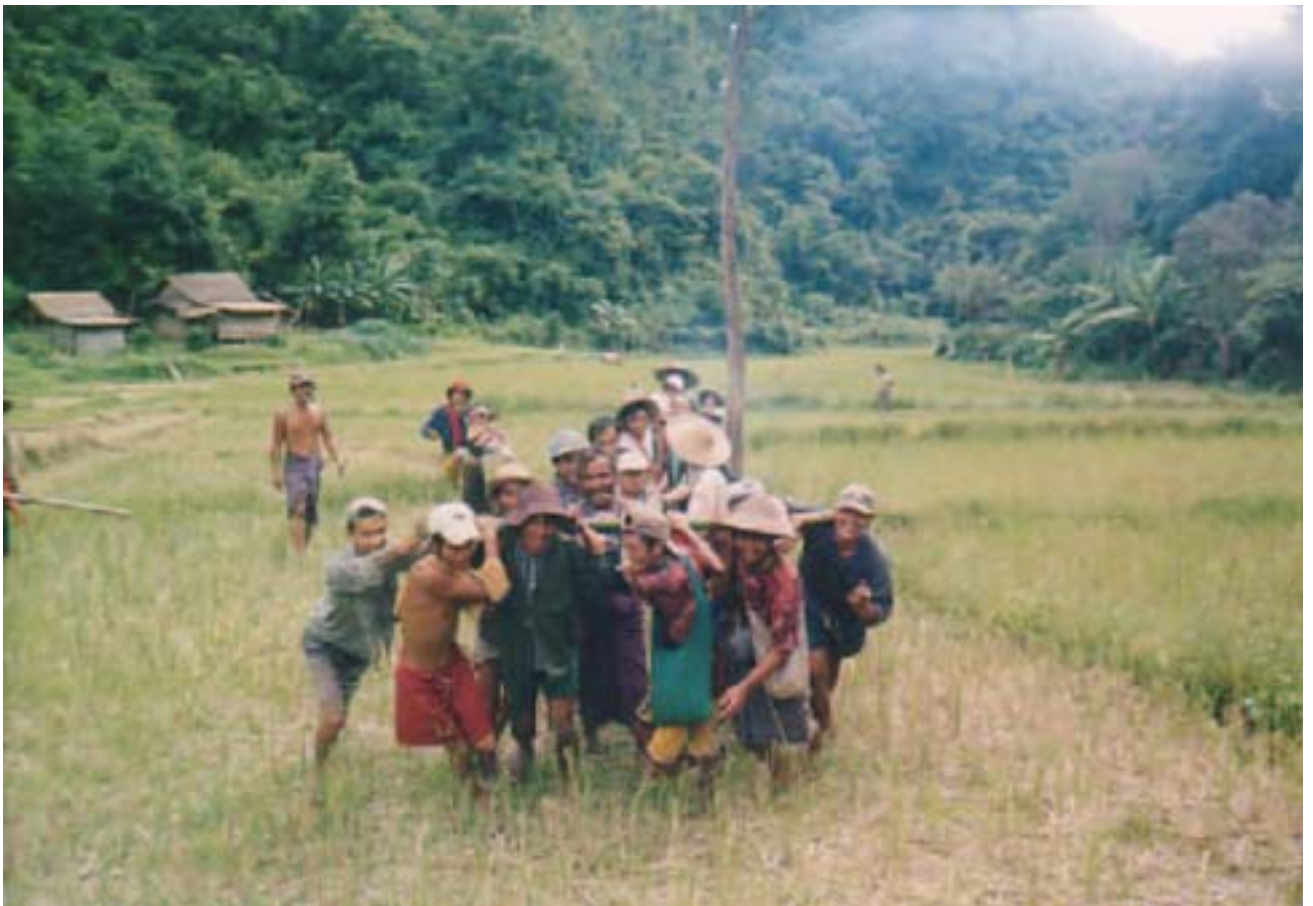
Construction on Self-Help: Transmission Lines
