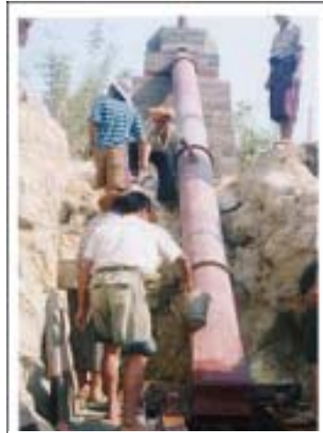
Penstock under Installation, Naung Bo
