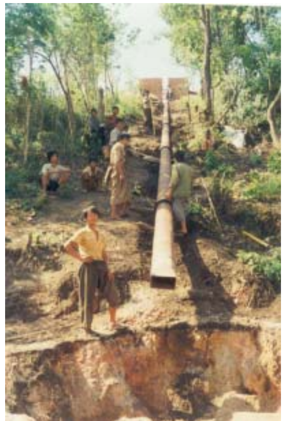
Construction on Self-Help: Waterways - Penstock (Pressure Pipe)
