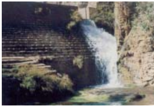
Sample of using existing structure Existing stone weir is used as intake.
