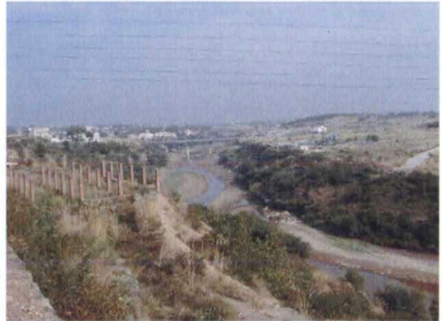
06 2.5km upstream of Confluence
