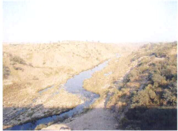
10 Upstream of Islamabad Highway Bridge
