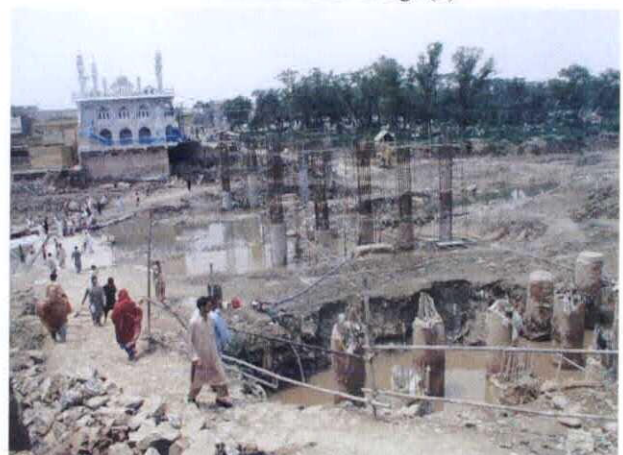
30 Pir Wadhai Bridge (1)
