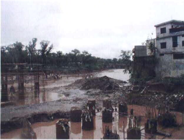
33 Flood Mark near Pir Wadhai Bridge (2)
