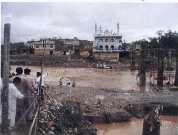
31 Pir Wadhai Bridge (2)
