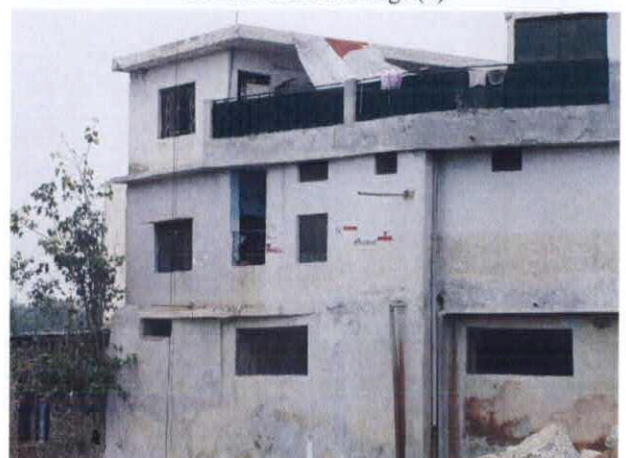
32 Flood Mark near Pir Wadhai Bridge (1)
