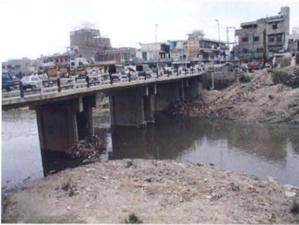
27 Gawal Mandi Bridge (1)
