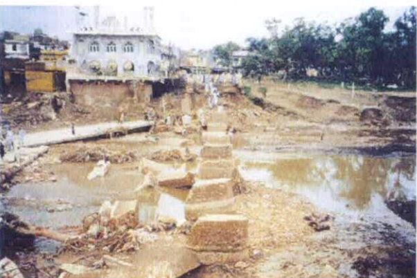
07 Pir Wadhai Bridge (3)
