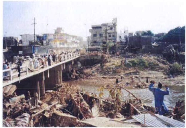
02 Gawal Mandi Bridge (2)
