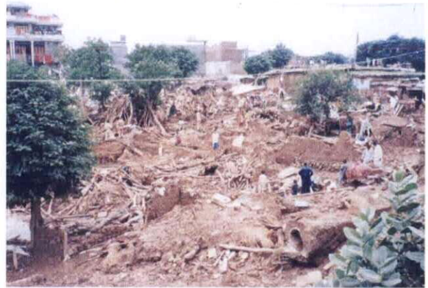
10 Bank Erosion and Collapsed Houses (1)
