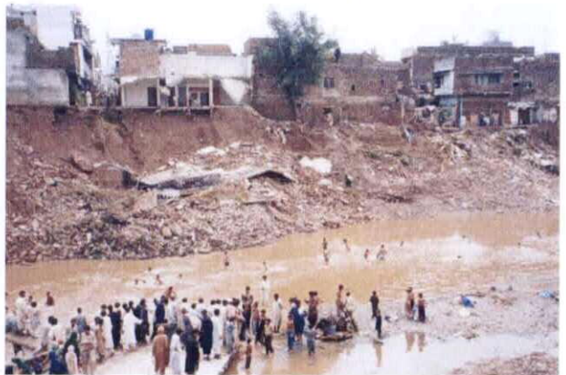
06 Pir Wadhai Bridge (2)
