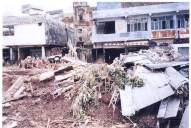
12 Bank Erosion and Collapsed Houses (3)
