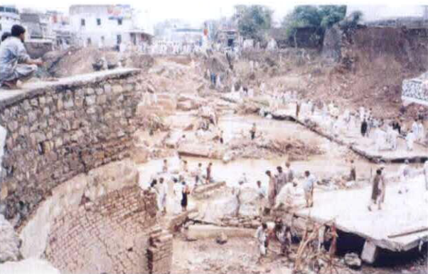
05 Pir Wadhai Bridge (1)
