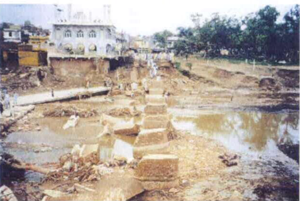
07 Pir Wadhai Bridge (3)
