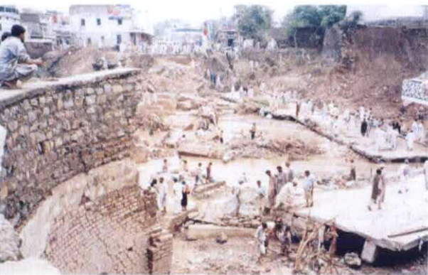
05 Pir Wadhai Bridge (1)
