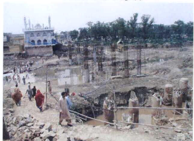
30 Pir Wadhai Bridge (1)
