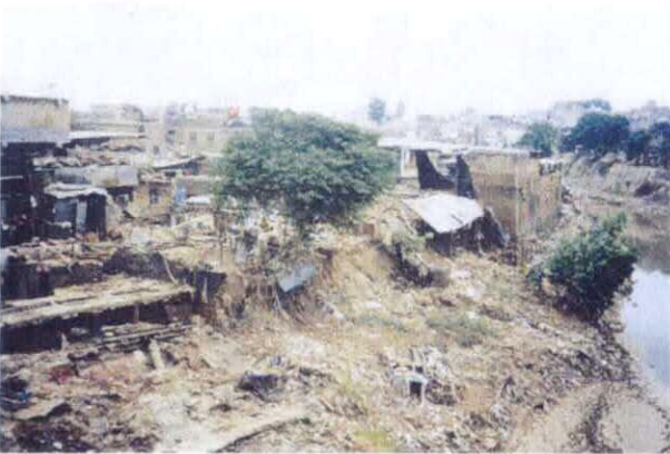
03 near City Sadar Bridge
