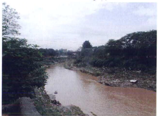
20 Downstream of Murree Bridge (2)
