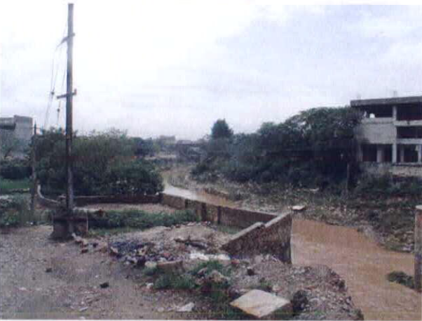
19 Downstream of Murree Bridge (1)
