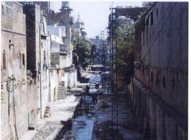
08 L3 Channel (80m upstream of Confluence)
