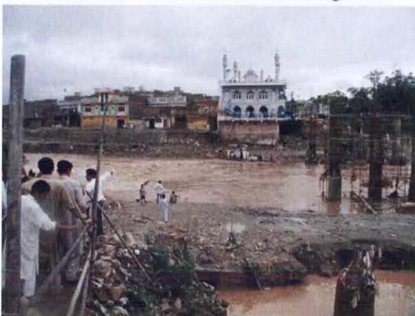
31 Pir Wadhai Bridge (2)
