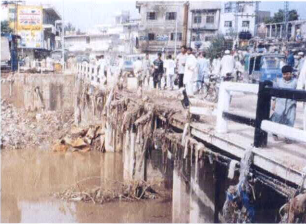
01 Gawal Mandi Bridge (1)
