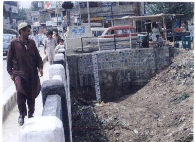
28 Gawal Mandi Bridge (2)
