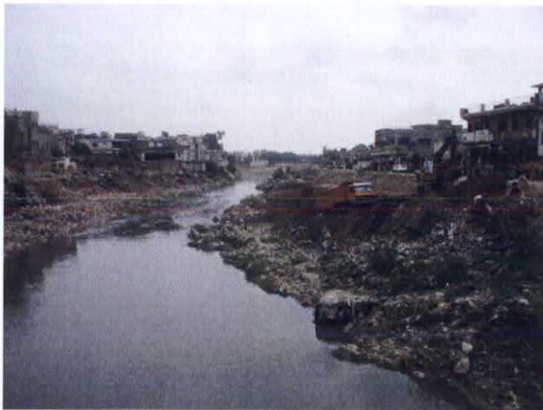
29 Downstream of Gawal Mandi Bridge
