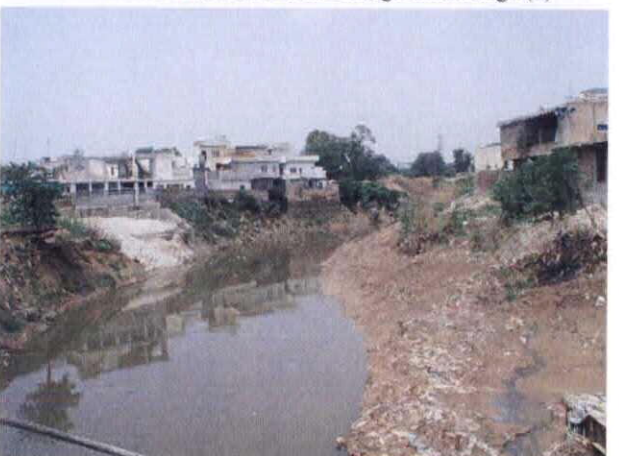
16 Upstream of Dohk Chiragh Din Bridge
