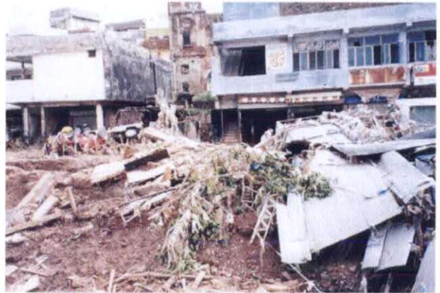
12 Bank Erosion and Collapsed Houses (3)
