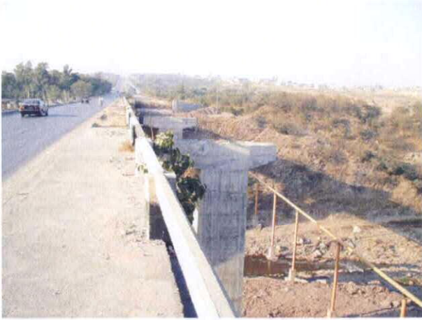
09 Islamabad Highway Bridge
