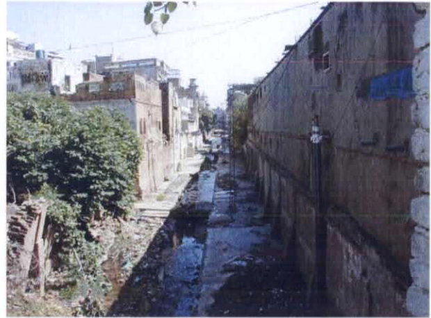
10 L3 Channel (120m upstream of Confluence)
