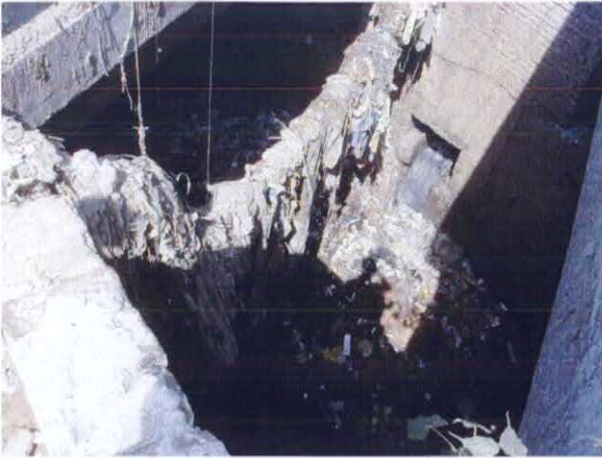
09 L3 Channel (100m upstream of Confluence)
