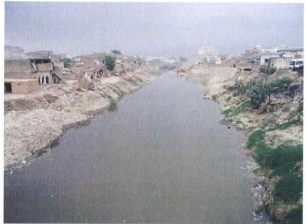
26 Upstream of Ratta Amral Bridge
