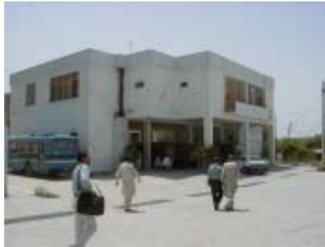
Main building of fire brigade
