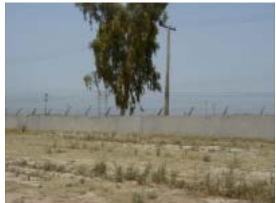
Fence of the double structure
