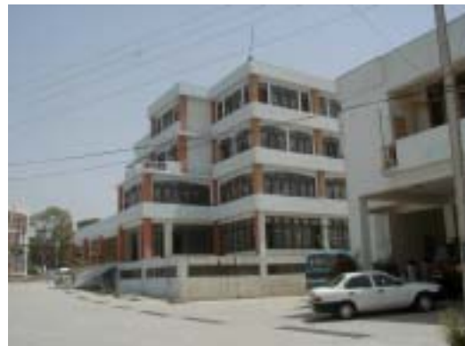
TMA's new building next to the Fire brigade
