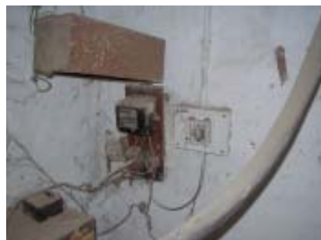
The expansion photograph of the siren Power supply equipment and switch of the siren
