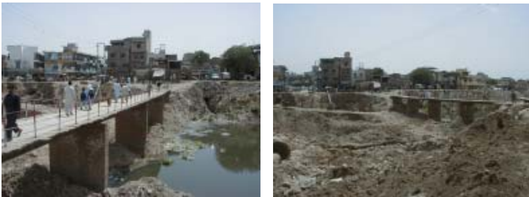
Gawal Mandi Bridge
