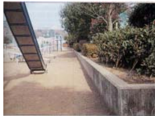
Flood Detention Wall at Public Open Space
