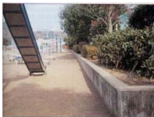
Flood Detention Wall at Public Open Space
