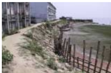
State of slope protection at the west bank
