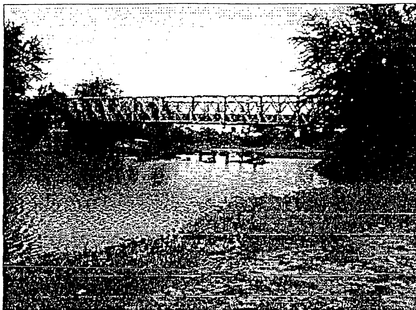
Photo-8 Temporary Bailey Bridge Along NR3
