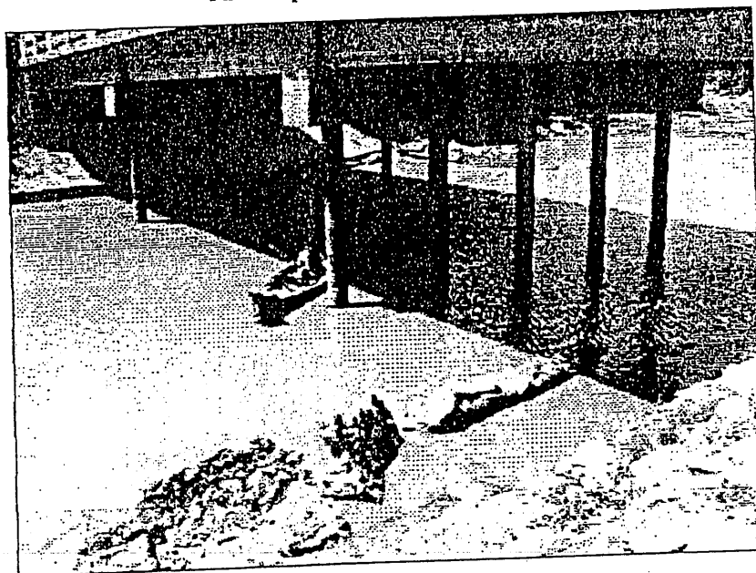
Photo-14 Serious Scoring at No.15 Bridge on NR6a
