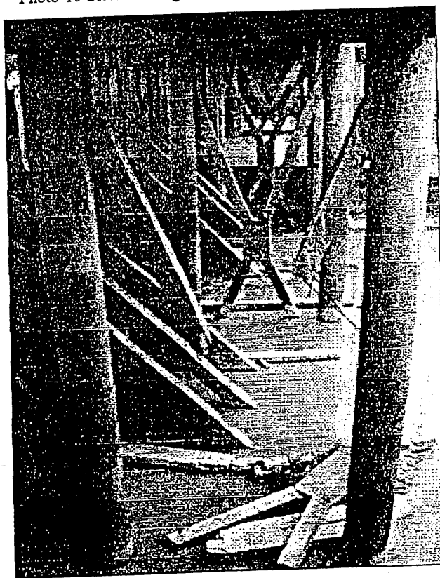
Photo-11 Collapsed substructure of Slakou Bridge NR3
