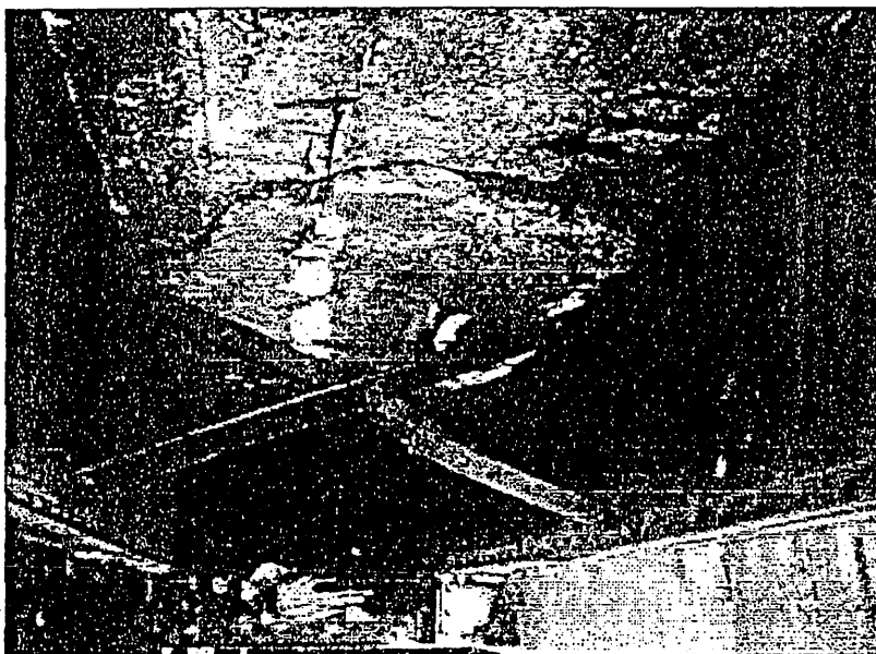
Photo-6 Ta Khamu Steel Truss, a deterioration on RC deck
