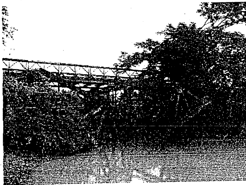
Photo-2 Bailey Bridge Constructed on Collapsed Bridge in Siem Reap
