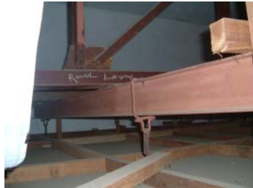
② Existing H-shape beam and connection
