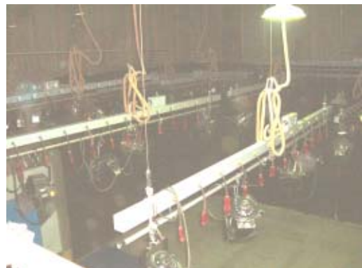
③ Existing lighting batten
