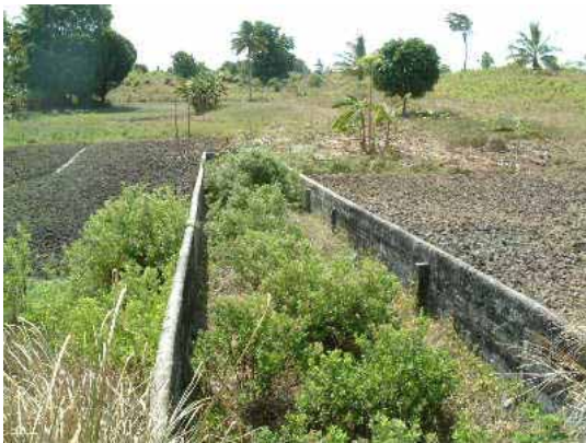
Constructed spillway
