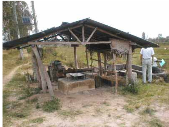
Damaged pump station
