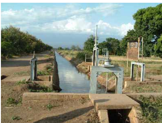
Canal system at existing Lower Moshi
