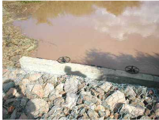
Gabion protection at diversion weir
