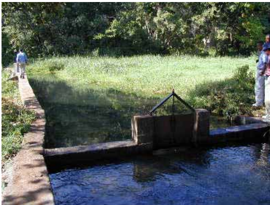
Diversion point at Mwananguruwe spring
