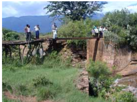
Proposed Intake Weir Site
