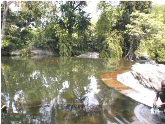
Mkindo diversion weir
