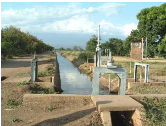
Canal system at existing Lower Moshi
