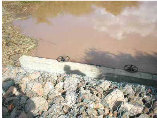
Gabion protection at diversion weir
