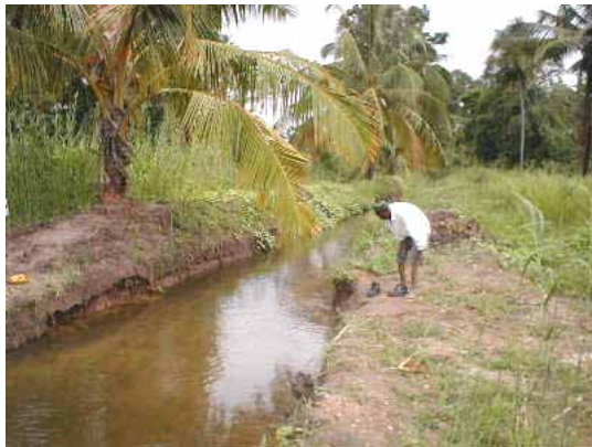
River diversion works
