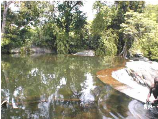
Mkindo diversion weir
