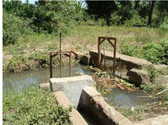
Existing canal facilities
