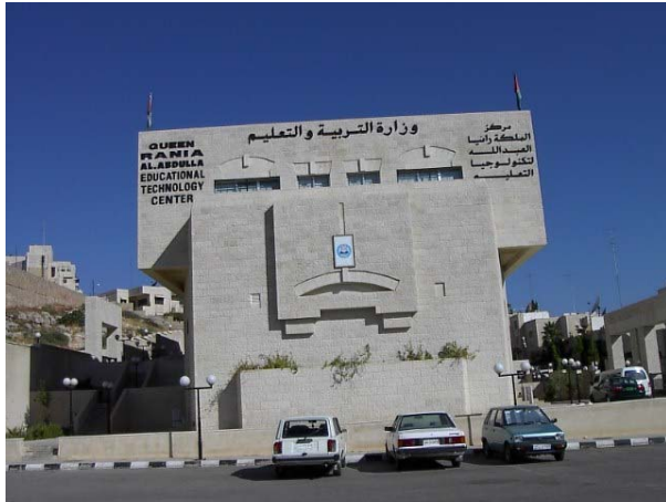
Learning Resource Center (Project Office)
