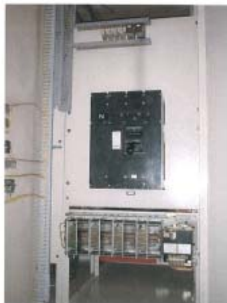
replacement of ACB on incoming panel
