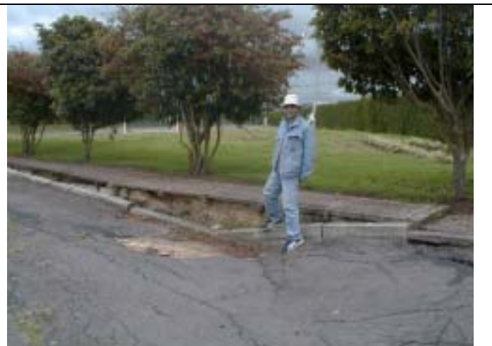
Depression of road in Siberia out of Bogotá City. Relation between depression and groundwater pumping was surveyed. However, there is no evidence between them so far.
