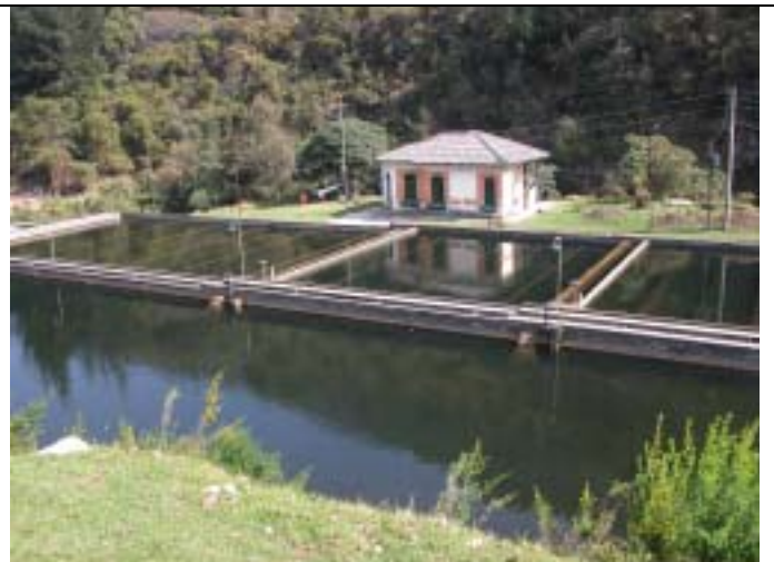
Siltation pond of Vitelma treatment plant. This site was selected for the implementation of the pilot project of artificial recharge.
