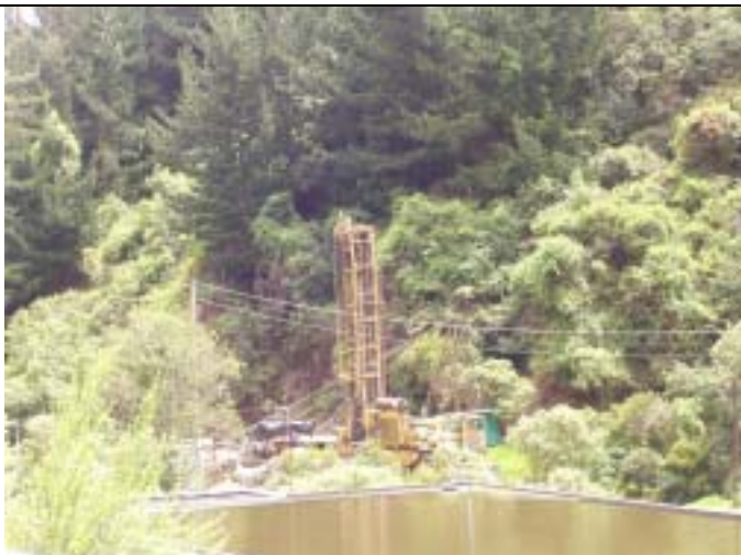
Situation of drilling well for artificial recharge in Vitelma (Pilot Study). This well proved high capacity of Guadalupe Formation at this site for artificial recharge (900m 3 /day).
