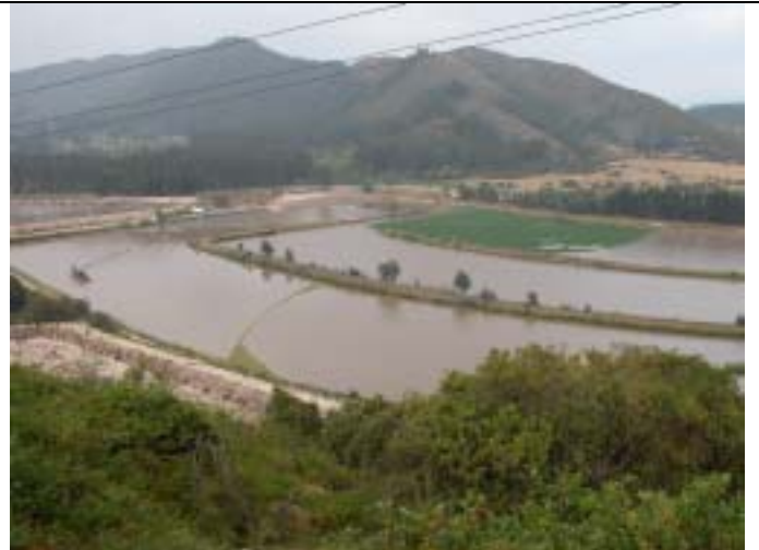
Tibitoc Purification Plant, other water source for water supply to Bogota City and neighbor municipalities. This plant takes water from North System including Bogota River. Intake rate can be reduced by groundwater development.
