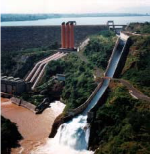
Figure-8 Karangates Dam Power Station
