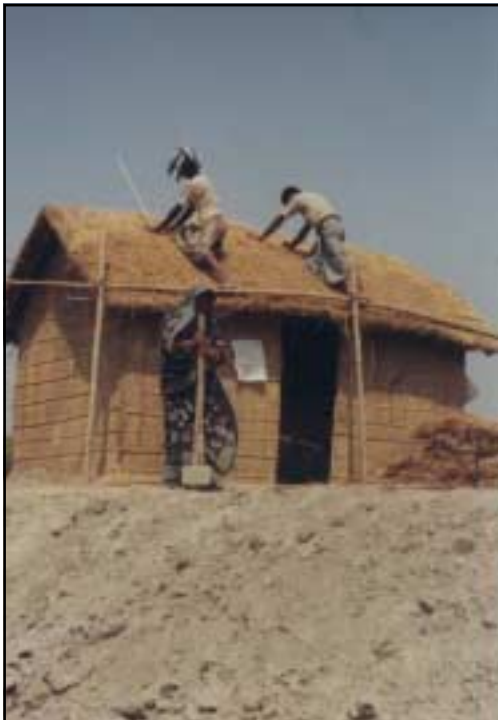
Reconstructing the House after Platform Raising
