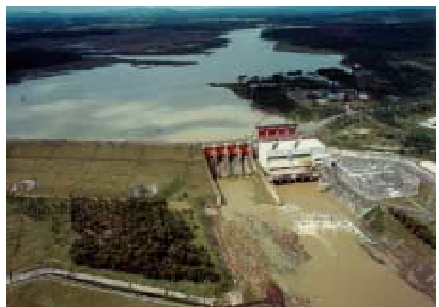
Figure-7 Wlingi Dam
