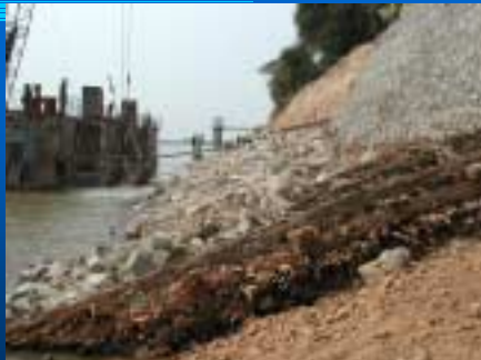
Covering the "SODA" Mattress with Stones
