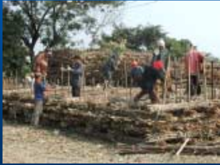
Constructing "SODA" Mattress
