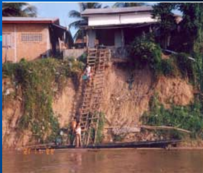
Houses being damaged by riverbank erosion in Vientiane Municipality
