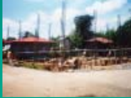
Construction of Baquero Norte Evacuation Site under Package III (September 2002)
