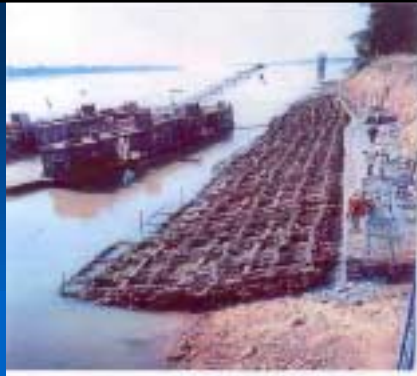
Installing "SODA" Mattress
