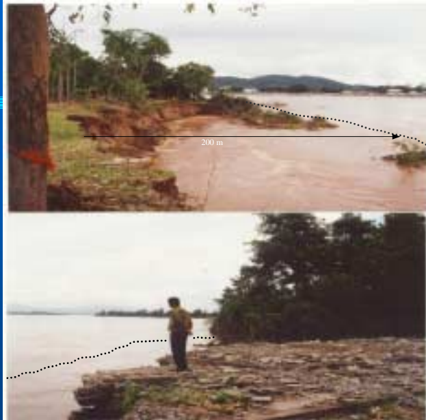
Serious riverbank erosion in Bokeo Province (August 28 2002)
