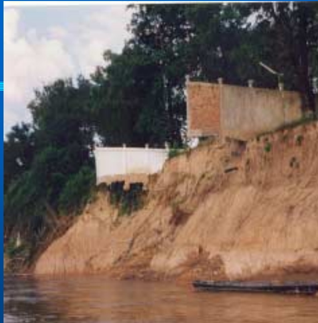
A factory destroyed by riverbank erosion
