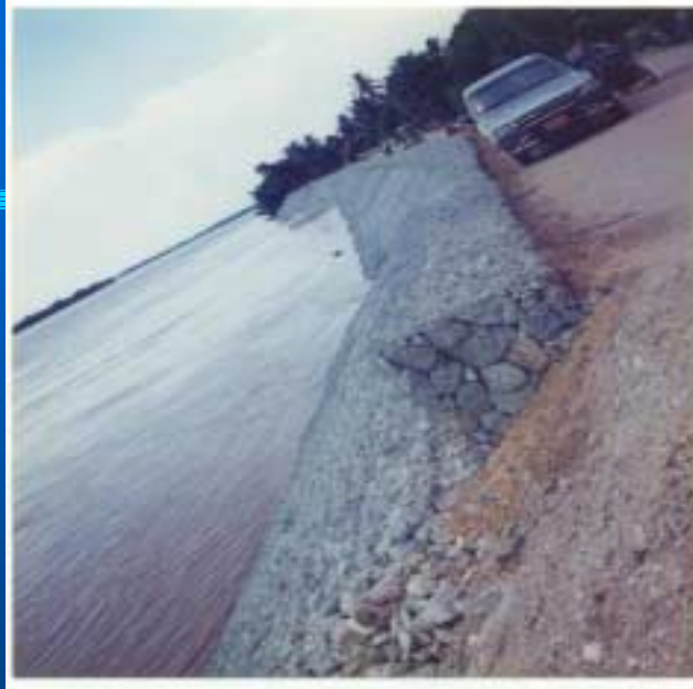
Past Riverbank Protection Works with Gabions
