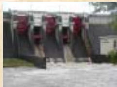
Shijushida Dam, controlling flood water
