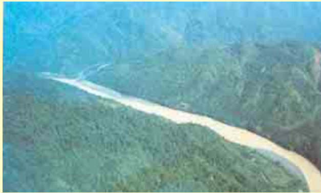
Agos Damsite (Looking Upstream)
