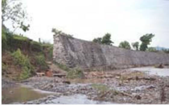
Existing Retaining Wall
