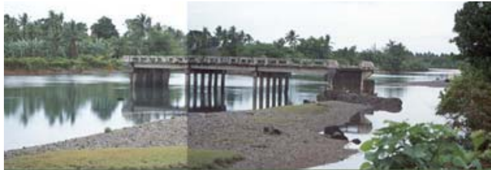
The bridge in Barangay Pinaglapatan, Infanta, Quezon Province
