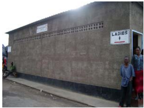
Photo5 Public Toilet by GCEP, George
