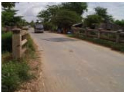
Existing Old Gate: Km50+040, Kampong Phnom Lied with Steel Plate on Road Surface & Slab
