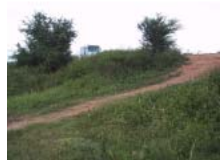
Embankment slope protected by vegetation
