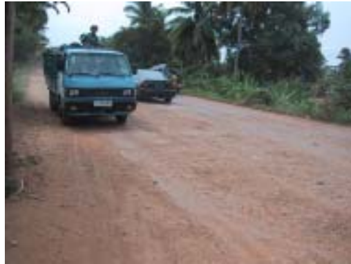
Destroyed pavement at Km 18+000-Km 19+000
