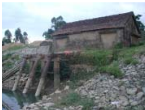
Nam Trung Pumping Station
