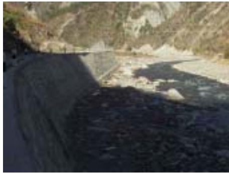
Dhulikel direction seen from Sta.13+800
