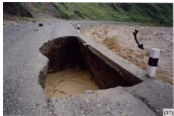
< Photo 3 > Type B-2: Scouring Depression of road surface
