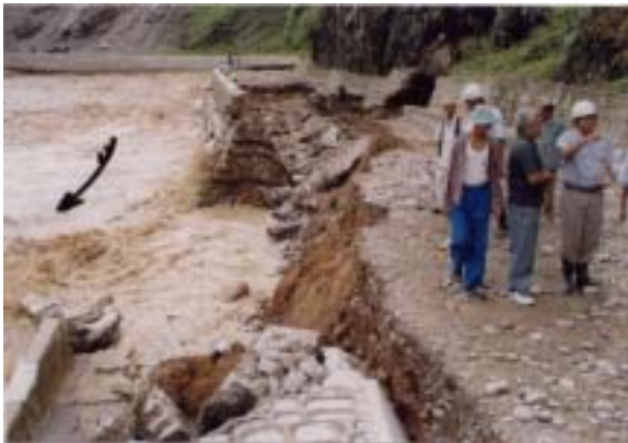
< Photo 7 > Type D: Destruction of revetment due to excessive hydraulic pressure
