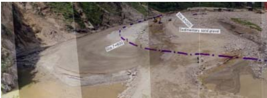
[No.24] STA.07+625 - 08+000 : Embankment washed away
