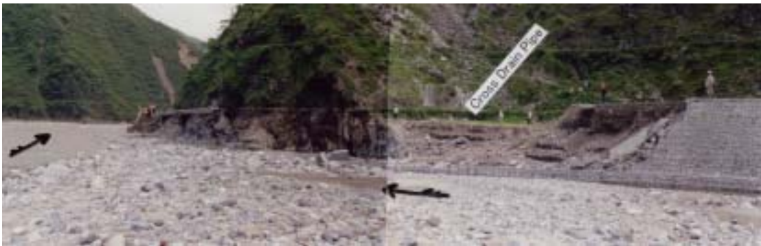
[No.24] STA.07+625 - 08+000 : Embankment washed away
