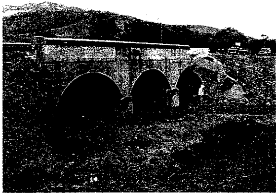
Photo 5.2.3 El Guayacan Bridge (Down stream side)
