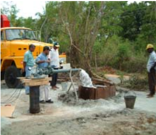
WRB engineers who conduct pumping test using donated submersible pump.
