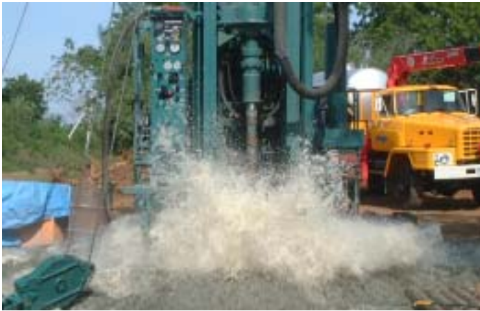
Groundwater is discharging from the well.
