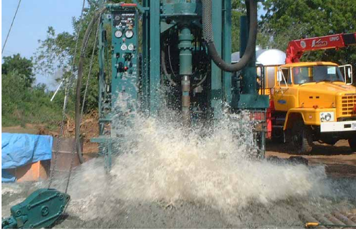
Groundwater is discharging from the well.
