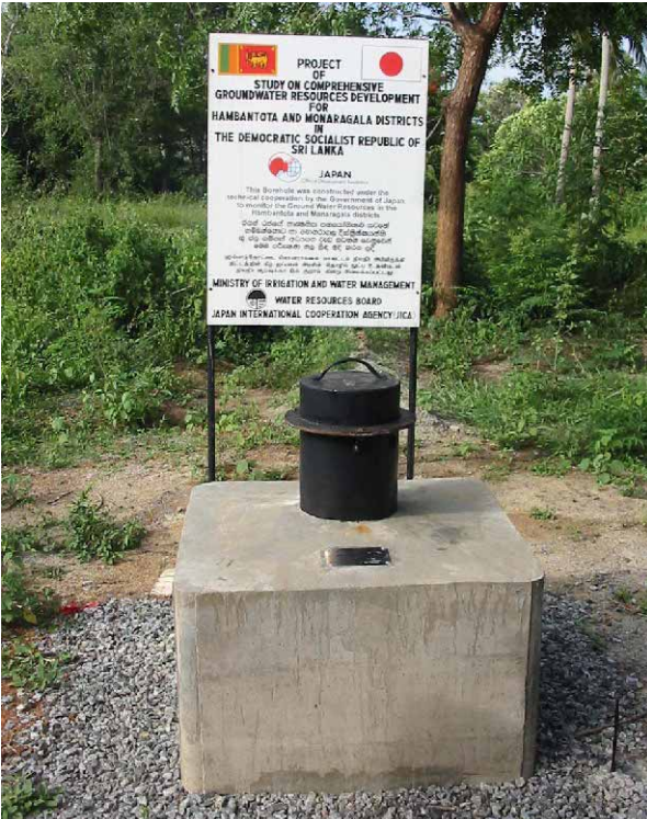
The completed test well and the signboard which shows the purpose of the well in three languages, Sinhalese, Tamil and English, made by WRB.
