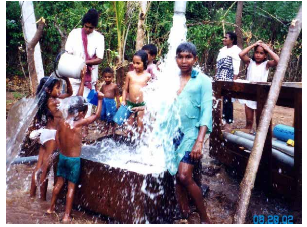
Residents are excited about the success of the well drilling. (Yarabowa)
