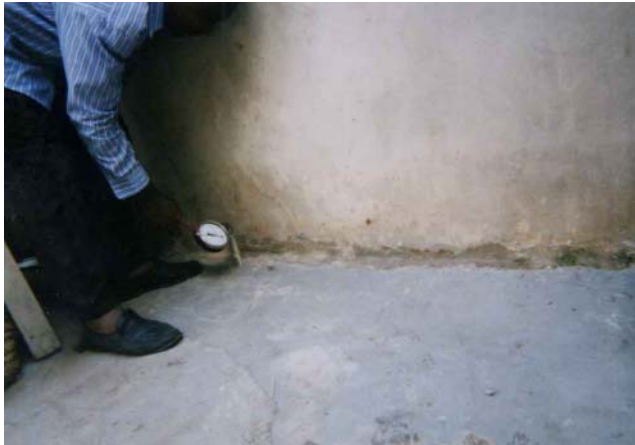
Pressure Reading in the Existing Pipelines
