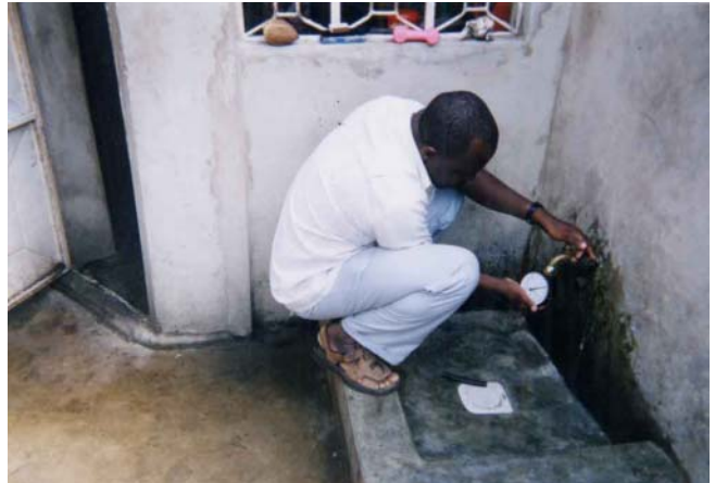
Pressure Reading in the Existing Pipelines
