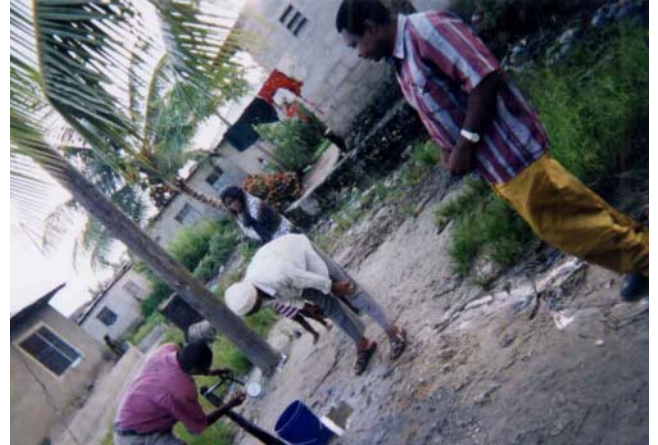
Pressure Reading in the Existing Pipelines
