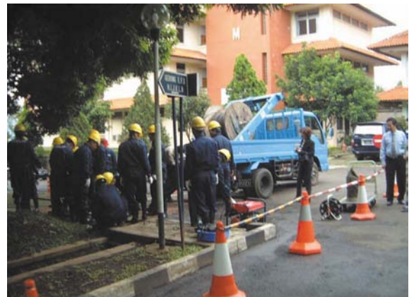
Local in-country training [Telecommunication Outside Plant Construction Technology]
