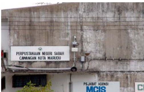
A 1.5m G.I. pole was erected at the side of the building where the Library is located.
