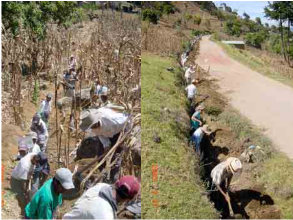
Mini Irrigation Plan : Installation of the Pipelines
