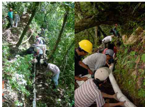
Rehabilitation Plan for Drinking Water System: Rehabilitation of the Pipelines
