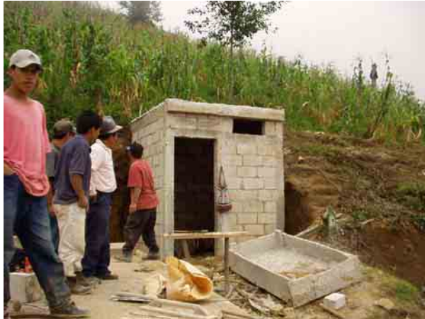
Water Quality Improvement Plan : Construction of the Shack
