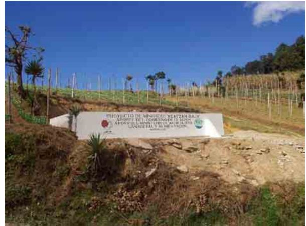
Mini Irrigation Plan : Construction of the Water Tank
