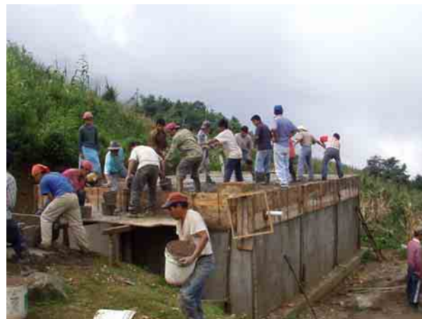
Rehabilitation Plan for Drinking Water System : Construction of the Water Tank
