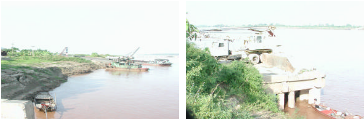
Photo 39.3.2 Upstream Scenery and Downstream End of Existing Facilities
