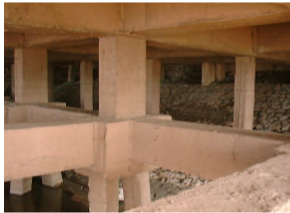
Beam, column without serious damage
