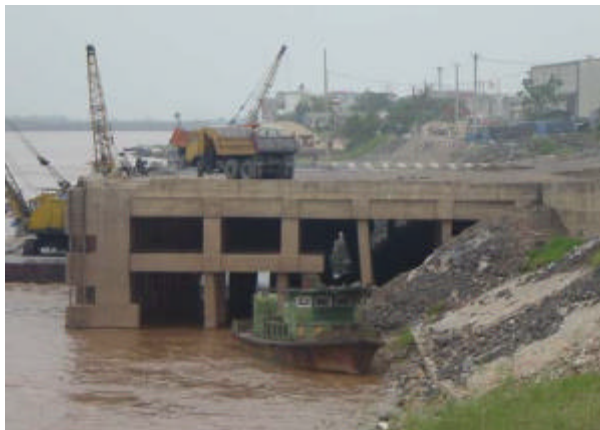
Side view of pier structure
