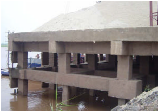
Side view of pier structure
