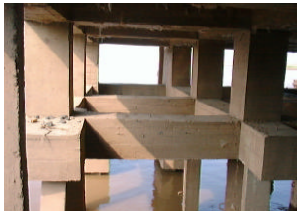
Beam, column with no serious damage
