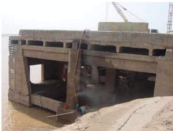
Side view of pier structure
