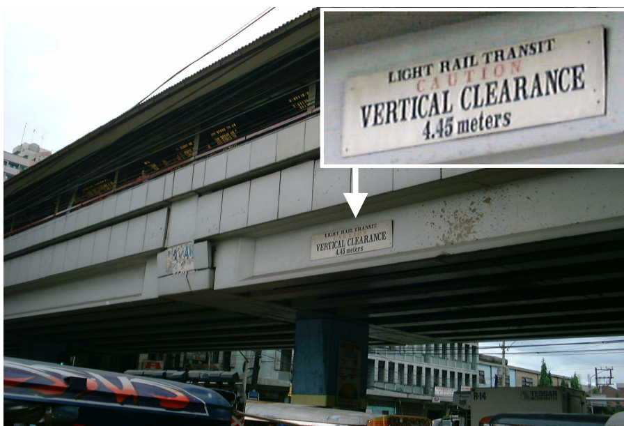
Figure 4.18 Caution Board at 5th Avenue Station of LRT 1
