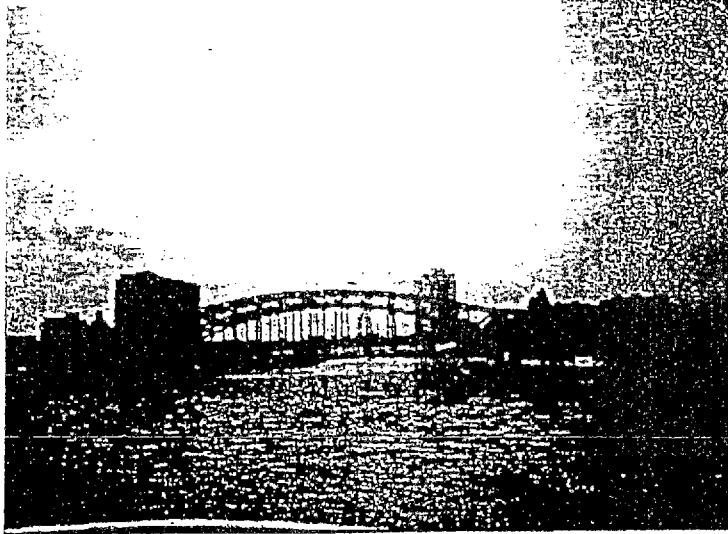
View of Quezon Bridge from the boat
