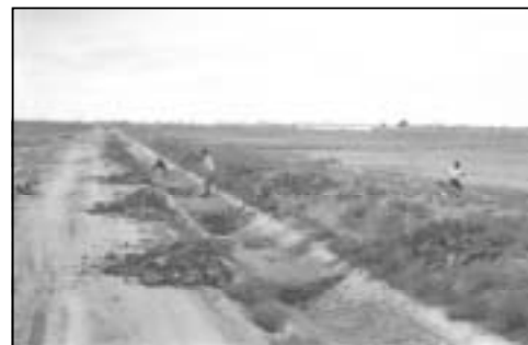
Scene of Silt Excavation from Irrigation Canal in Banavar I&D Scheme
