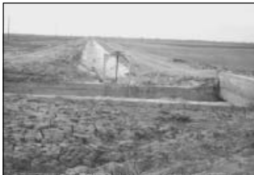
Division Work for 2ndary Canal .
