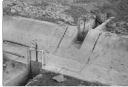
Divisin Work for Tertiary Canal
