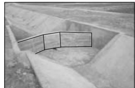
Desilting Basin Along Canal
