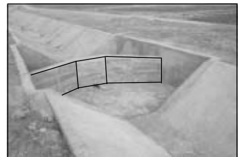
Desilting Basin Along Canal
