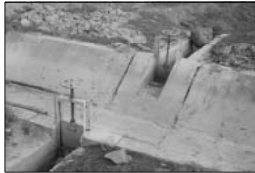
Divisin Work for Tertiary Canal
