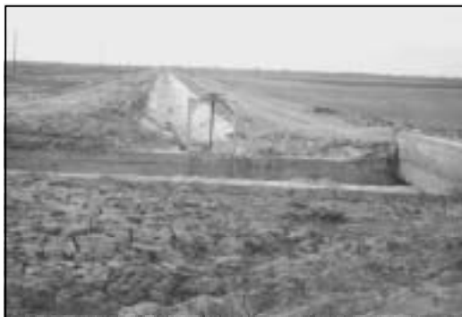
Division Work for 2ndary Canal .
