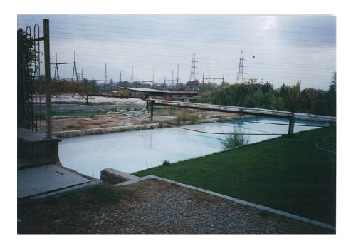
8. The renewed equalizing lagoon (Esfahan); vertical pipes in the lagoon for mixing by air bubbling.
