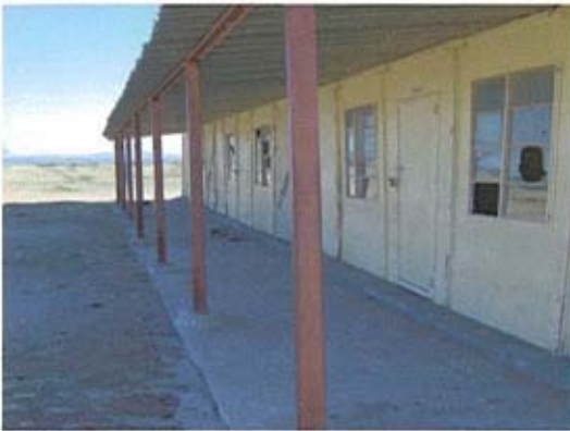
Structural distortion with no brace, weak for gale force
