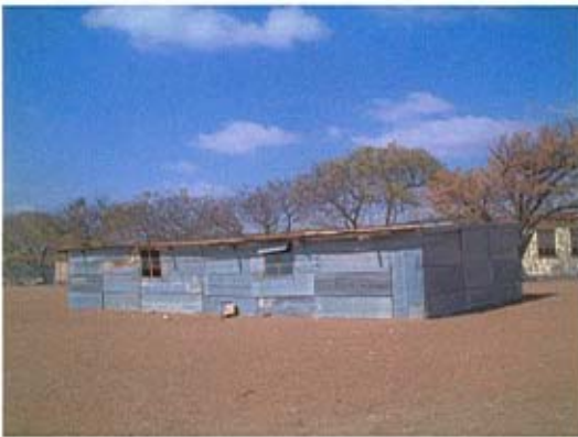
Structural distortion with no brace, weak for gale force
