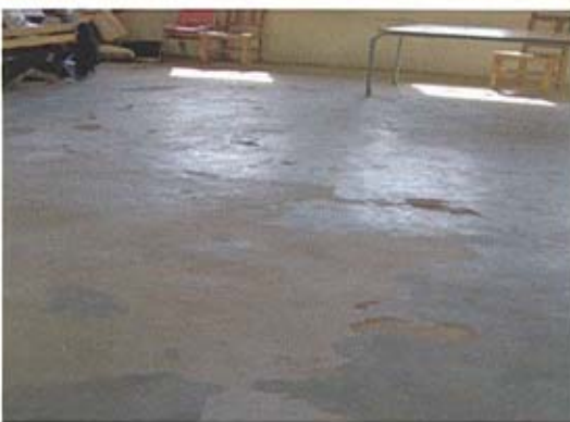
Damaged floors by floated mortar and hair cracks on mortar rendered walls could be repaired unless structural defects
