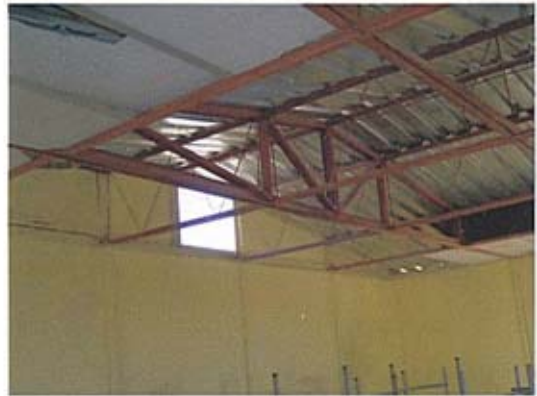
Significant defect of component panels-wall and ceiling
