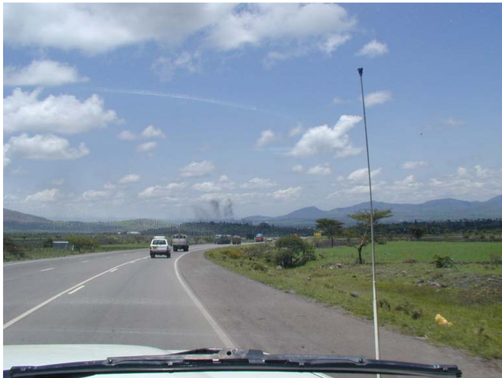
Photo No.14: The Suburban Trunk Road Shoulder Condition of Optical Fiber Laying Route between Addis Ababa (Nefas silk) and Nazareth
