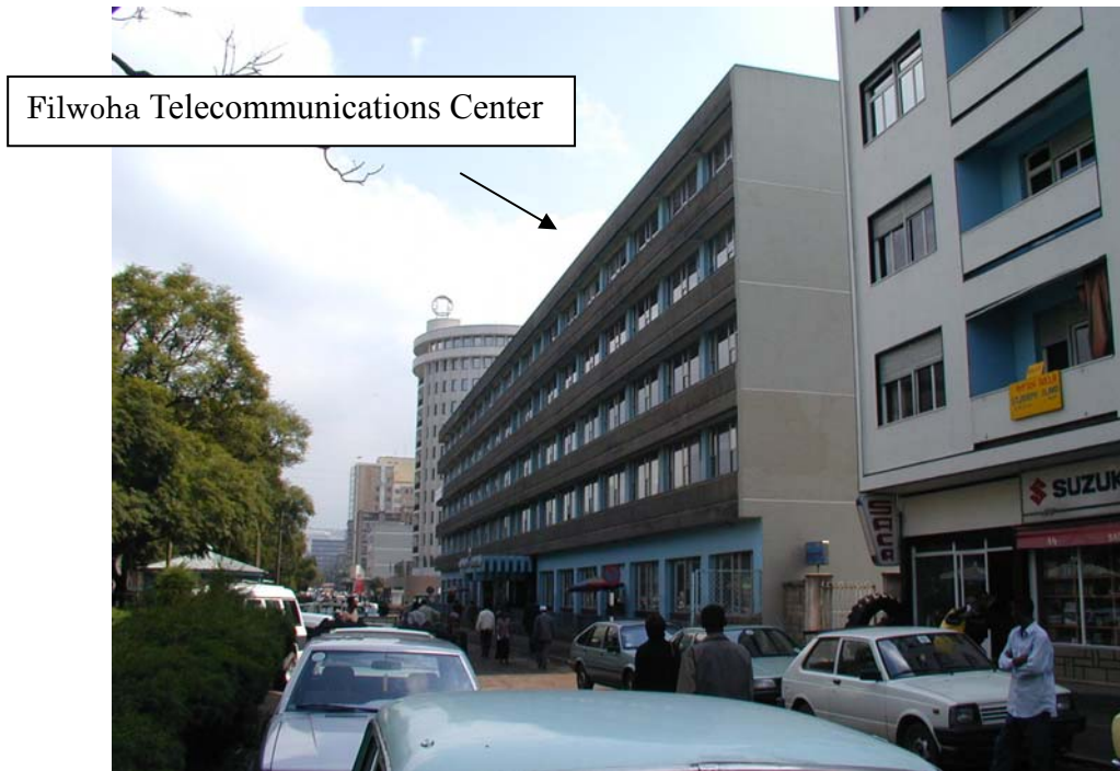
Photo No.5 : Addis Ababa-Filwoha Telecommunications Center Building
