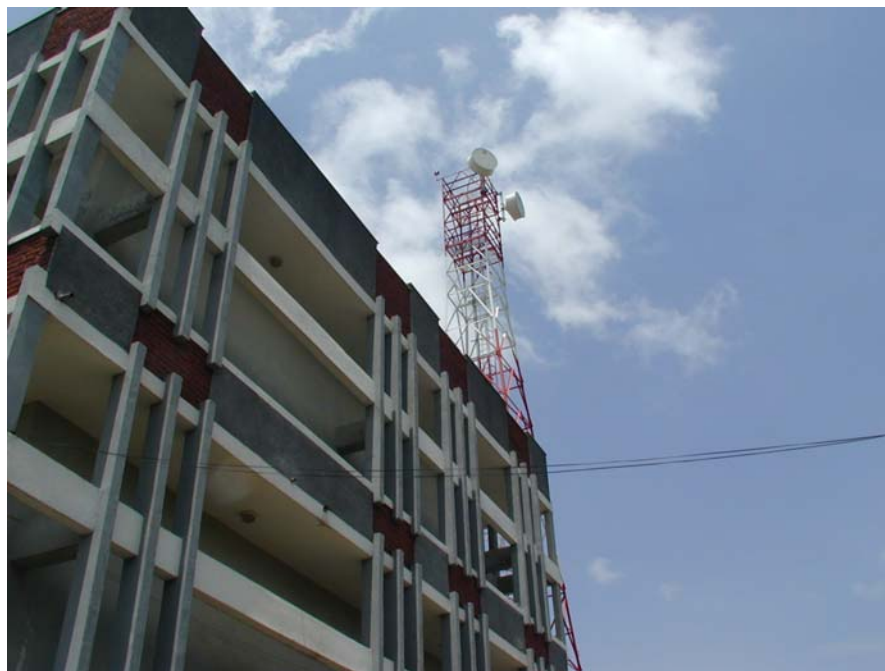
Photo No.6 : Addis Ababa--NEFAS Silk Telecommunications Center Building
