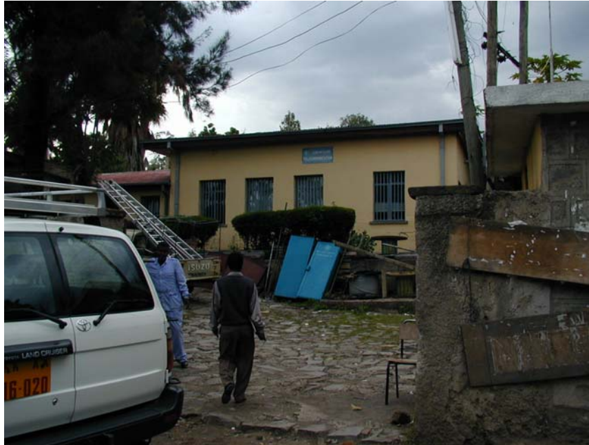
Photo No.8 : Debre Zeit Telecommunications Station Building Main Gate
