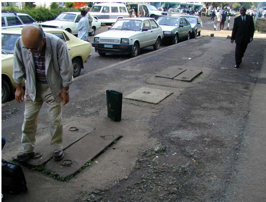
Photo 1: Duct Survey in Front of AA- Filwoha Telecommunications
